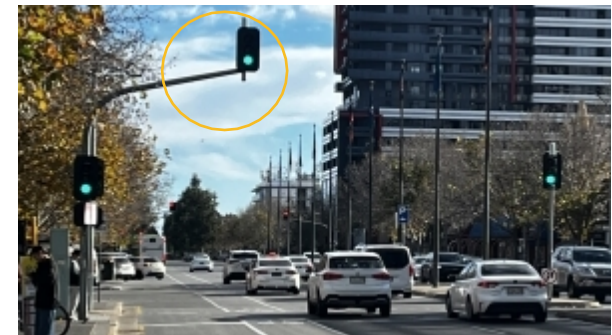
Example of a mast arm (circled) – to be added to some PACS to improve visibility of signals
